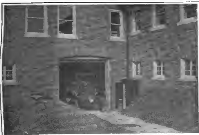
ENTRANCE TO GARAGE IN BASEMENT UNDER MAIN BUILDING.
